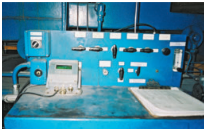
Vaisala's DMP248 Transmitter monitors dewpoint in a sintering furnace.
