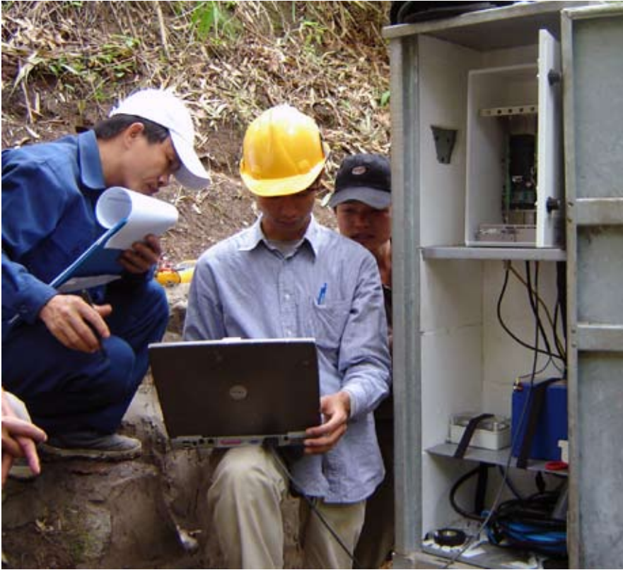
Site Acceptance Testing in progress.
