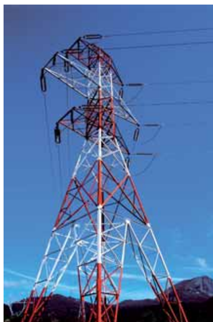
The efficiency of the power lines is a function of wind speed and direction.
